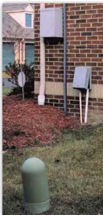
Tom Ped is the answer to these types of MDU problems.
