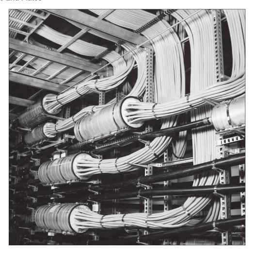
The ARMADILLO Stainless with Fire Retardant Drillable End Plates is a custom system designed to upgrade existing vault closures without disturbing the splices or interrupting the service. This system can also be used for new construction
